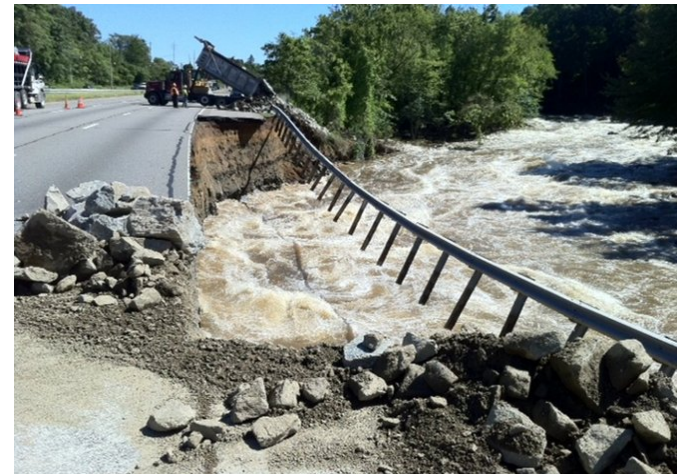
NJ 287 collapse from Hurricane Irene
