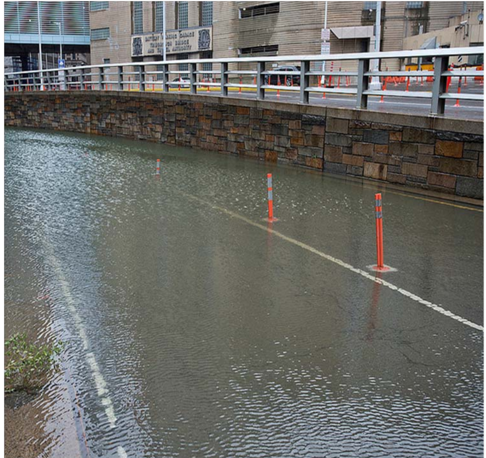
Photo: Flooding of the Hugh L. Carey Tunnel in NYC due to Hurricane Sandy. Source: MTA
